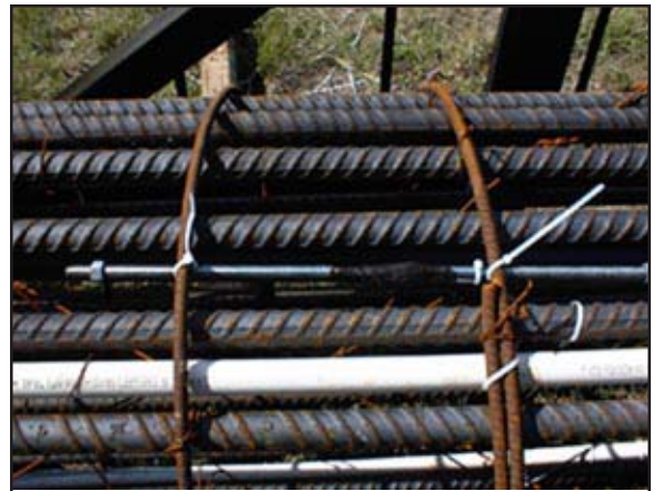
Fig. 5 Strain Bars installed on rebar cage
