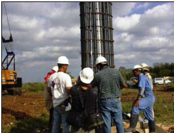
Fig.1 Installation of instrumented cage
